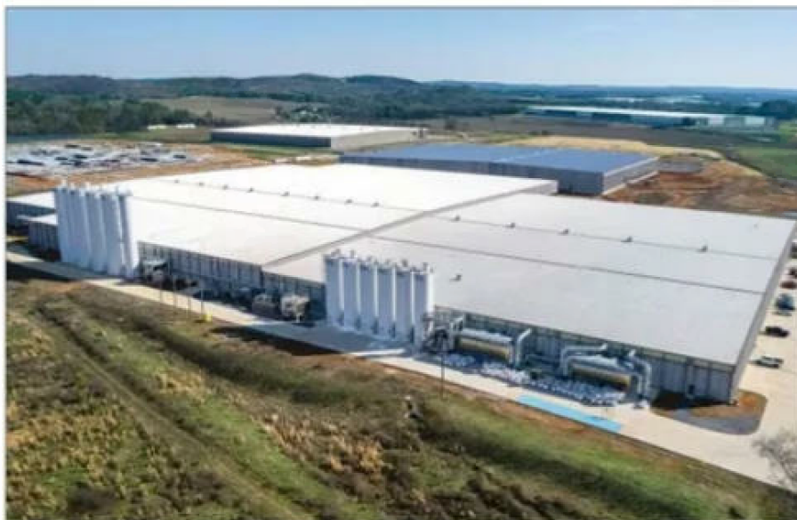
CFL's Calhoun, Georgia facility.
